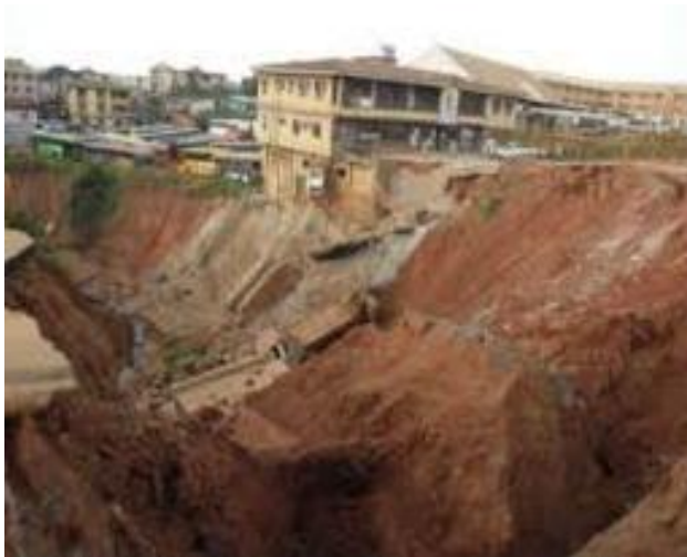
EROSION SITE Threatening Residential Buildings
